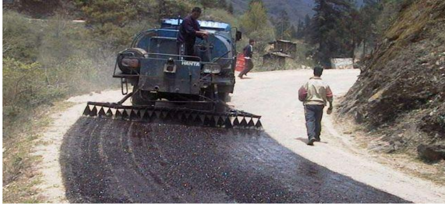
Spreading binder material
