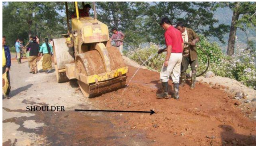
Construction of shoulders
