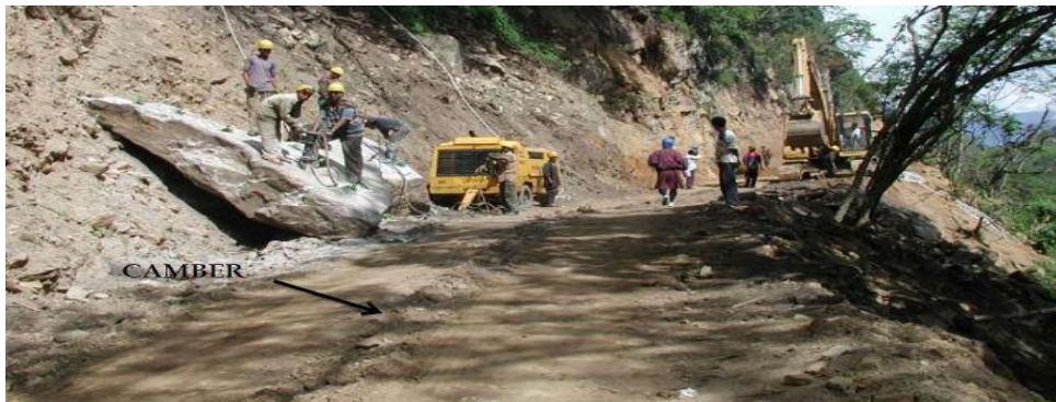
Sub grade preparation
