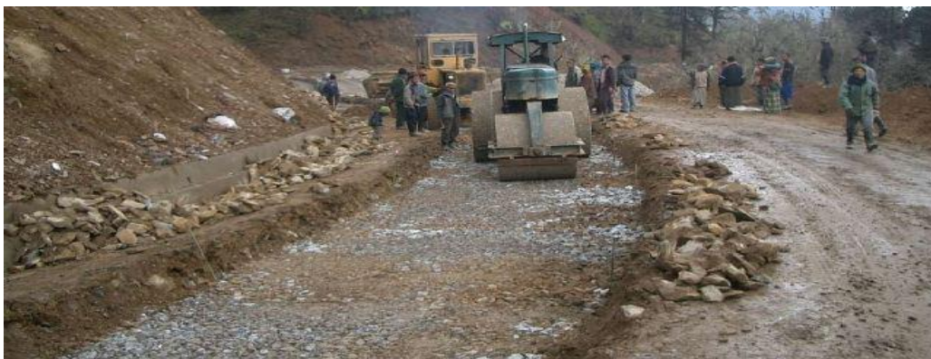
Roller Compaction
